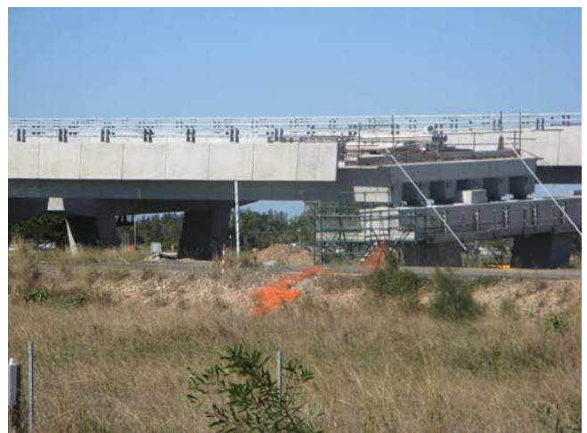
Teven Bridge, part of the Ballina bypass project.
